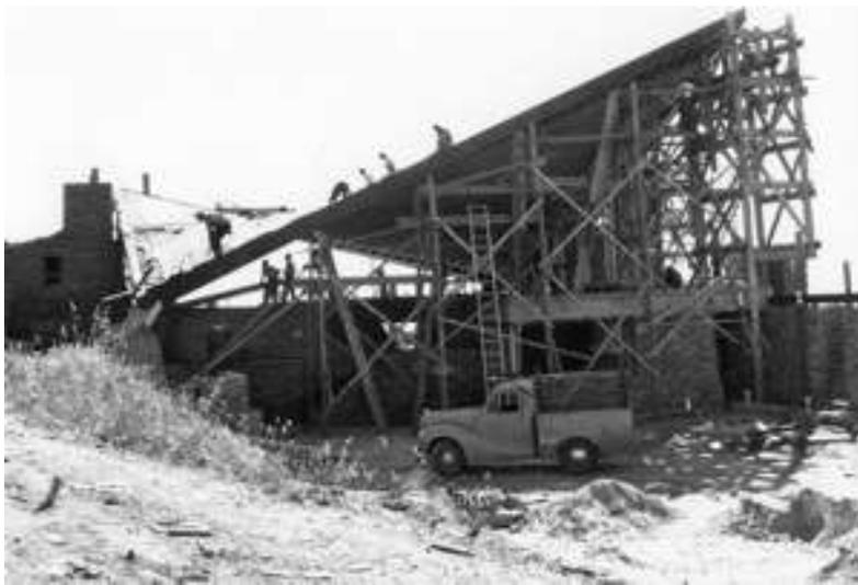
The roof itself was quite easy to construct and covered in copper sheeting with yellowwood for the ceilings. The problems came in with the anchoring to the supports and here they had trouble with the engineers who were brought in. The architect felt that their calculations were wrong and devised his own scheme – which did not go down well! However when the roof
